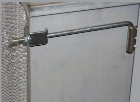
Swing bolts and equi-bearing clamps ensure an airtight filter to frame flange seal.
